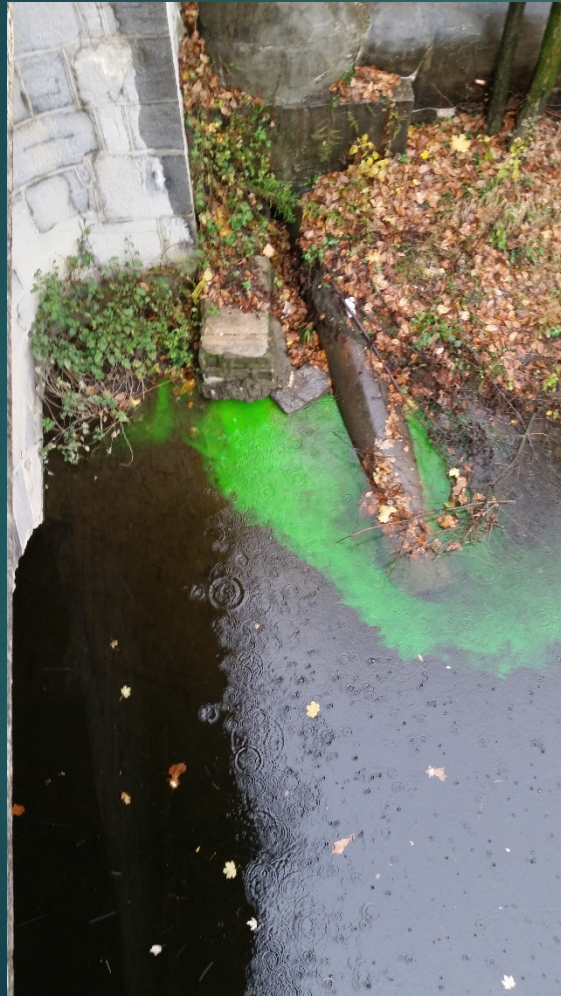
BEFORE PIPE LINING
