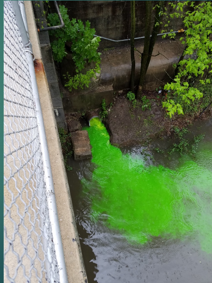
AFTER PIPE LINING
