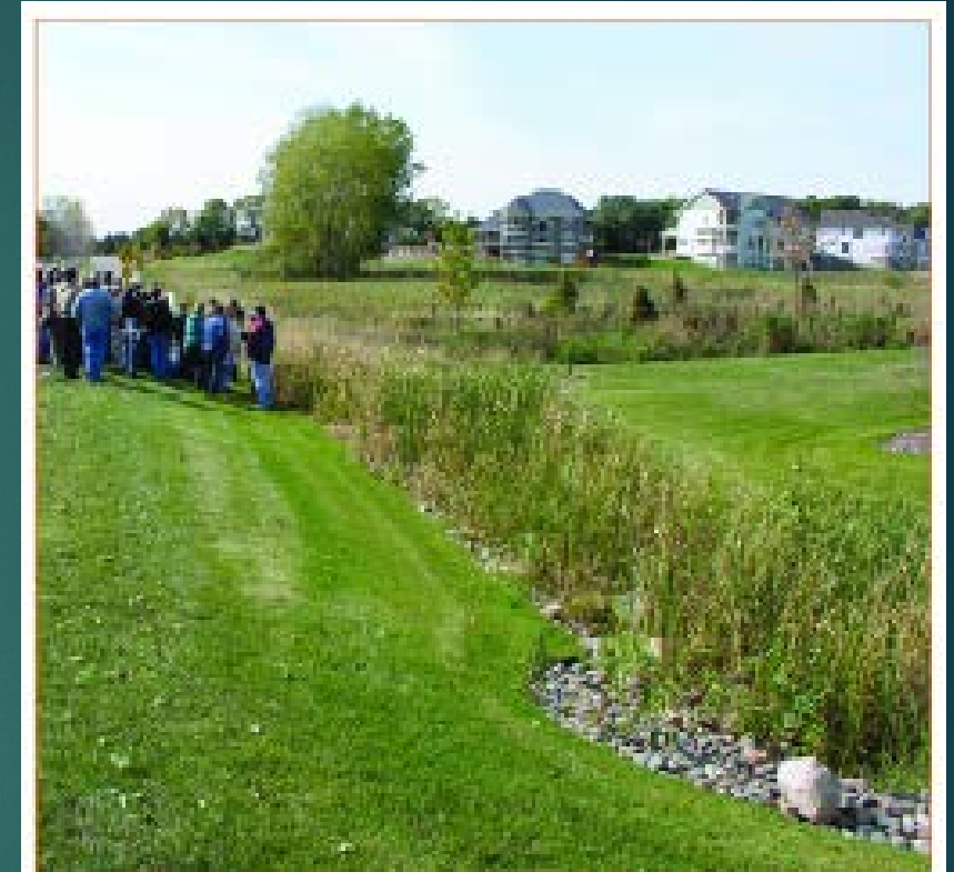
A road ditch can serve as a bio-swale. The rock trench and wetland vegetation are notable features, along with the natural drainageway in the background that serves as a bio-swale for residential runoff.
